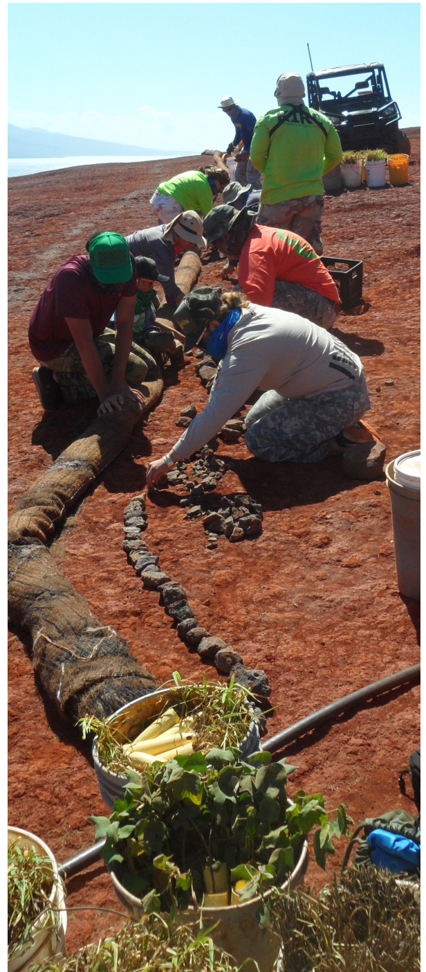
Kamehameha Schools Kumu building wattles in the DOH 4 work site above Hakioawa.
